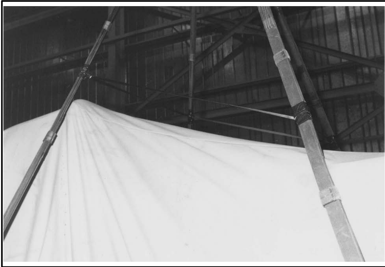
Figure 2-8 Deadman Ties Installed
