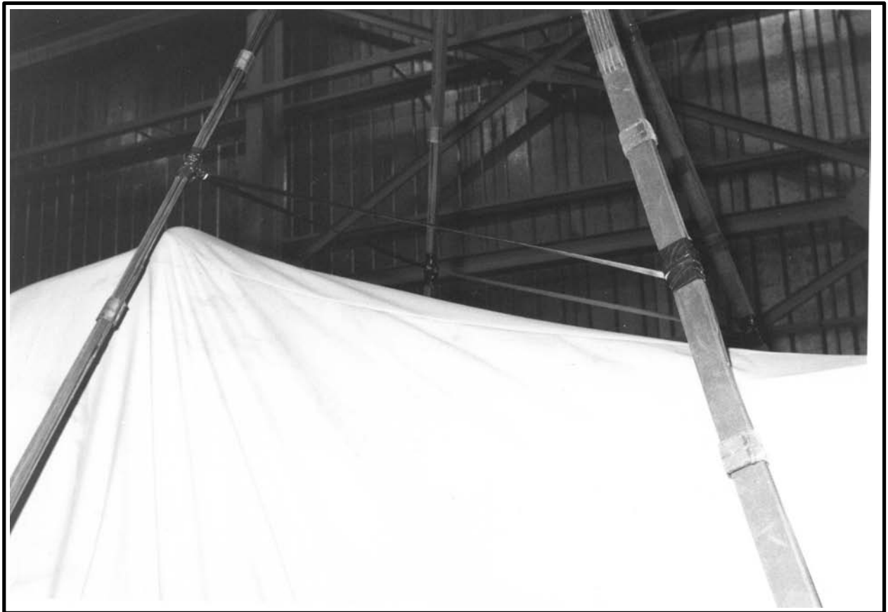
Figure 4-24 Deadman Ties Installed
