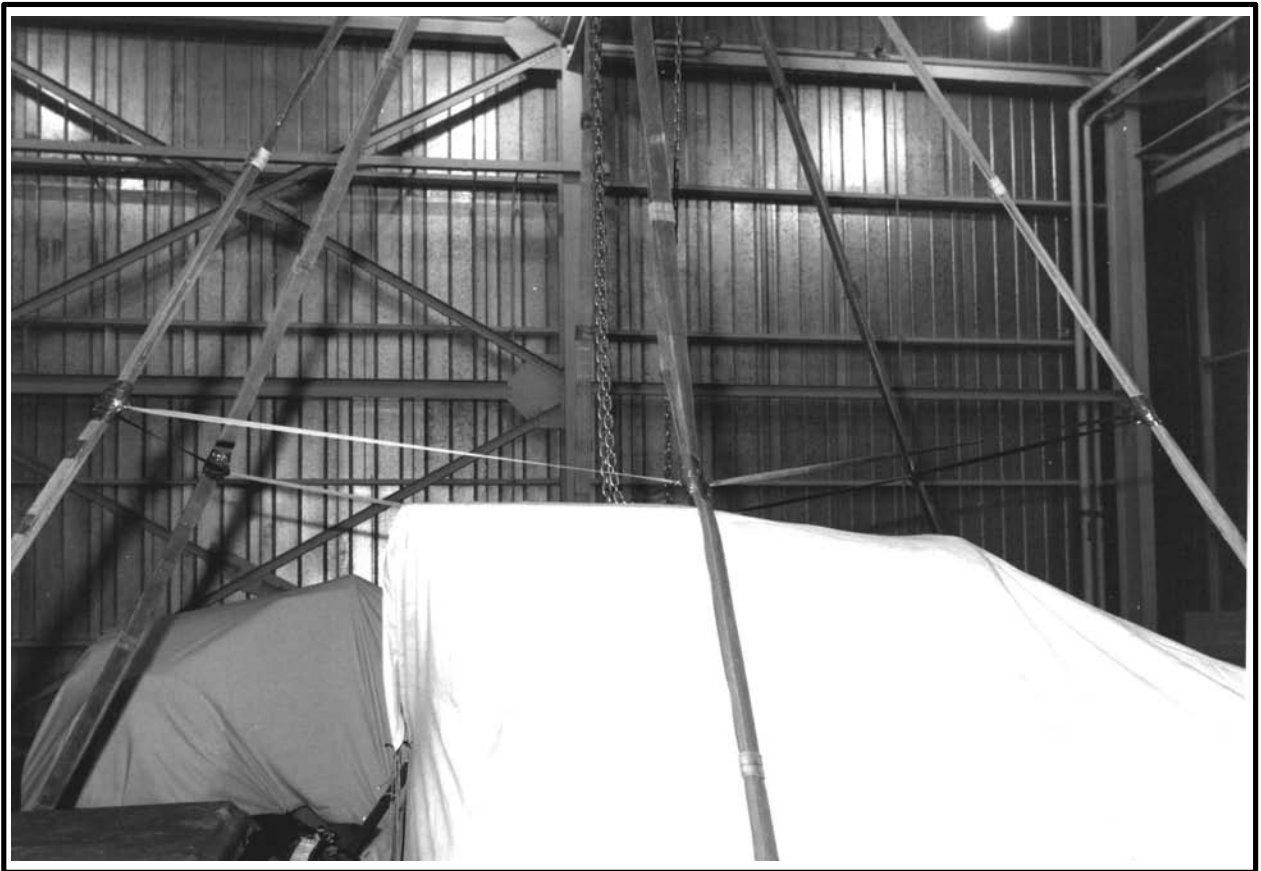
Figure 8-17 Deadman Ties Installed
