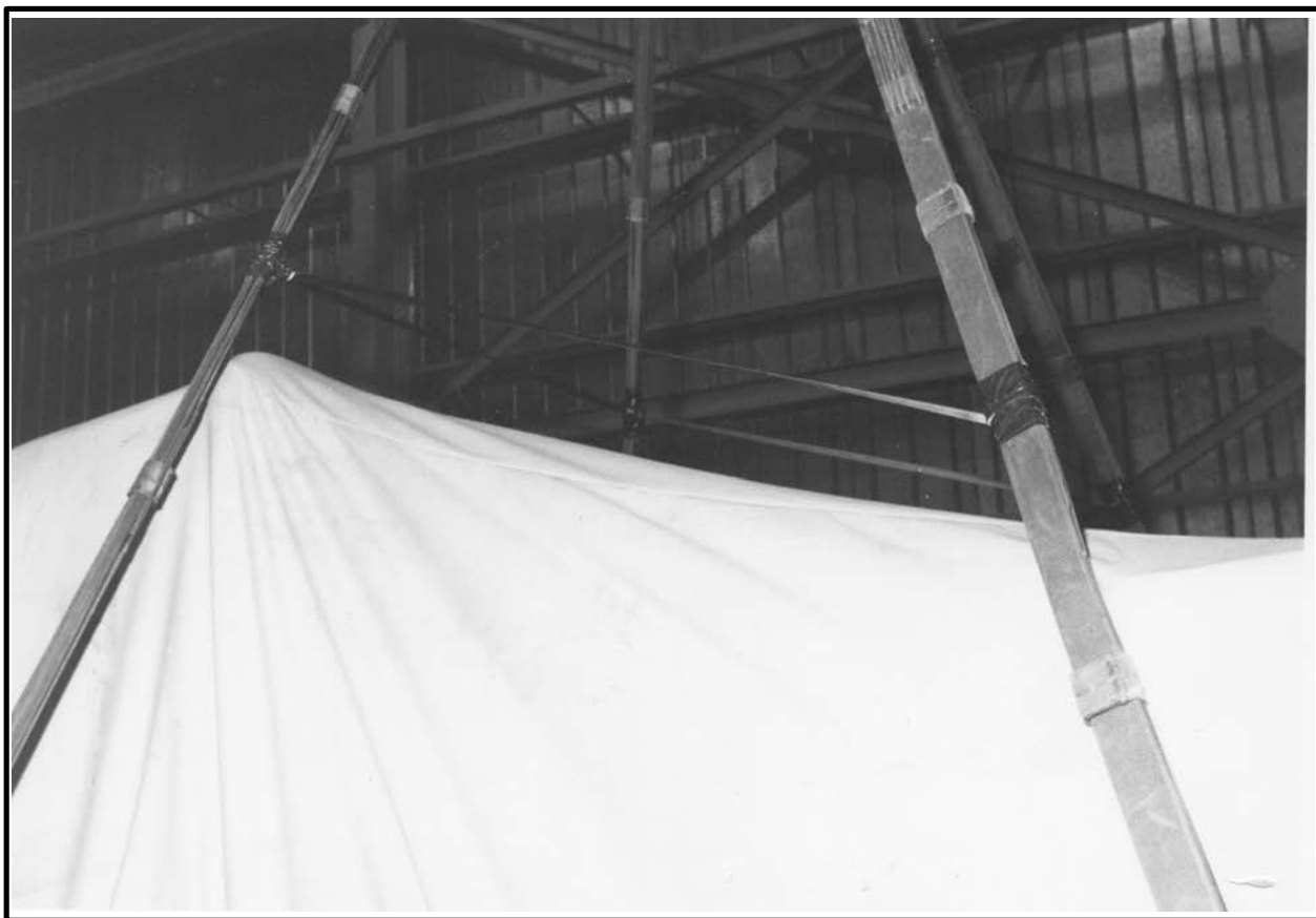
Figure 6-32 Deadman Ties Installed
